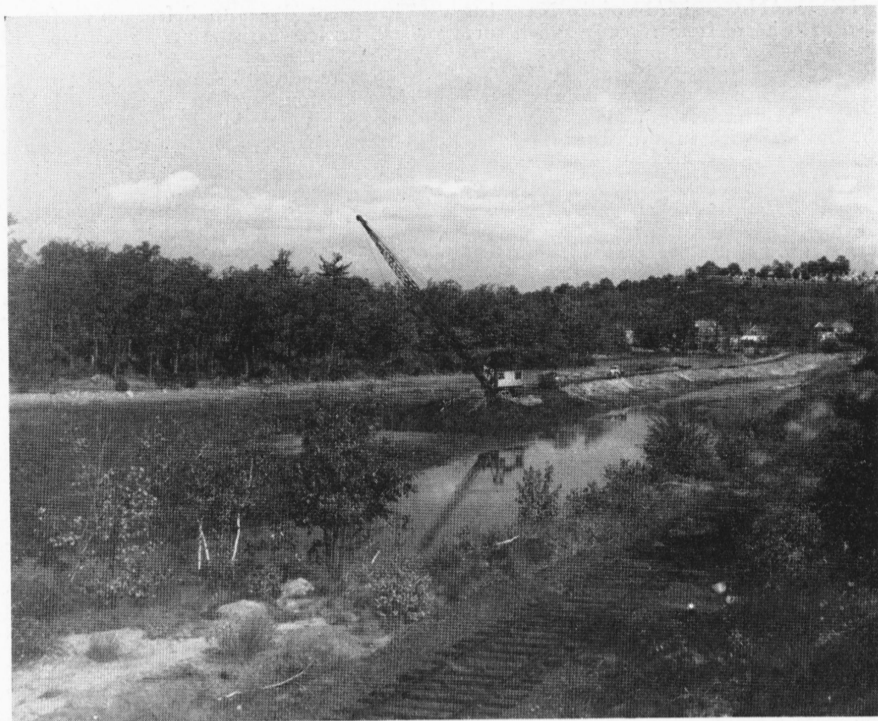
From an especially-built roadway extending out into the Brass Mill Pond, this dredging shovel is removing silt and accumulated debris from the basin of the pond in the first cleaning since it was built in 1915. After a portion is dredged out, the road is scooped up behind the shovel. The Brass Mill Pond is a Scovill-owned reservoir, east of Hamilton Park.
